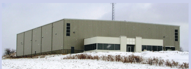
FRONT OF BLDG. (WEST SIDE), & NORTH SIDE
