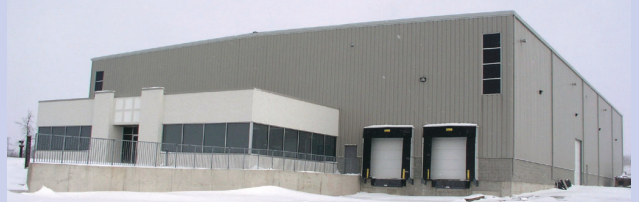
FRONT OF BLDG., (WEST SIDE), W/ (2) DOCKS, & SOUTH SIDE
